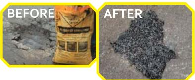
PAR by IMCO° is specifically designed and engineered to permanently repair potholes in asphalt. PAR can be installed in any weather condition, including wet, freezing and extreme heat, and is ready for traffic immediately after repair.
